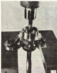
PRESSING OUT THE OUTER DRIVE SHAFT
