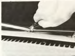
INSTALLATION OF WEATHER STRIP
