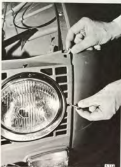
REMOVAL OF SCREWS, FRONT PANEL
