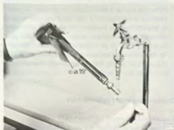
HOLDING THE FLAP VALVE IN POSITION
