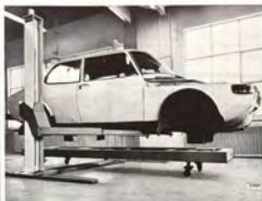
MOUNTING THE CAR IN THE JIG
