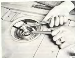
DISCONNECTING THE FUEL LINE
