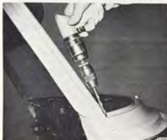
DRAINING HOLES ARE DRILLED
