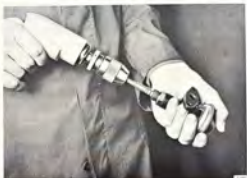
CLEANING THE INLET OF THE EGR VALVE
