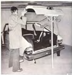
LIFTING AWAY THE TRUNK DOOR
