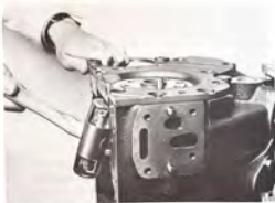
REMOVING THE GABLE PLATE
