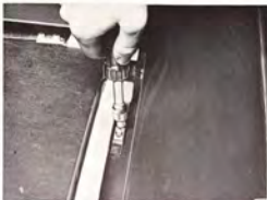
THE FASTENING IRONS WITH PLASTIC WEDGES ARE INSTALLED
