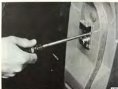
ADJUSTING THE STRIKER PLATE
