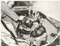
SEPARATING THE INNER UNIVERSAL JOINT
